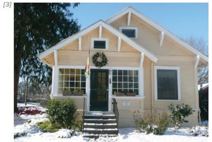
Roof Forms. [1] Roof pitches less than 4 over 12 are prohibited and roof forms will consist of more than a single large roof form [2] Gables shall be decorated with window(s), trim or a vent [3] Roof eaves will project at a minimum 12 inches.
