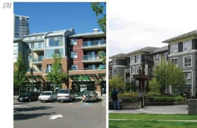
Large Building Elevation. [1] The front elevation of buildings with street-facing facades greater than 500 square feet should carve the building face into smaller, distinct planes, which can be accomplished by [2] incorporating a porch or dormer into the wall plane or [3] recessing the building a minimum of 2 feet over 6 feet.
