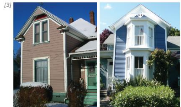
Windows. Windows are character-defining and should reflect the characteristics of existing windows in the historic district [1] Windows should be vertically-oriented [2] Windows should cover a minimum of 15% of the street facing façade [3] Windows should have an architectural feature such as a decorative header or cap, continuous trim, and a projected or articulated window sill.
