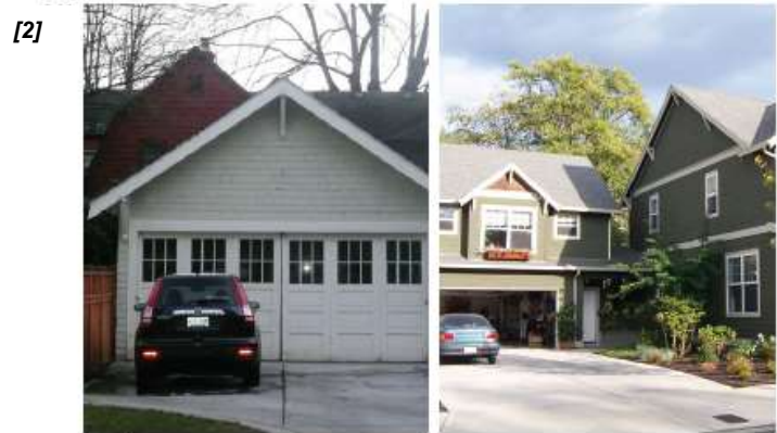
Accessory structures. [1] Detached, covered accessory structures should not exceed a maximum lot coverage of 25 % of the site as they are secondary uses and should not detract from the primary use [2] They can be used to house an attached dwelling unit.
