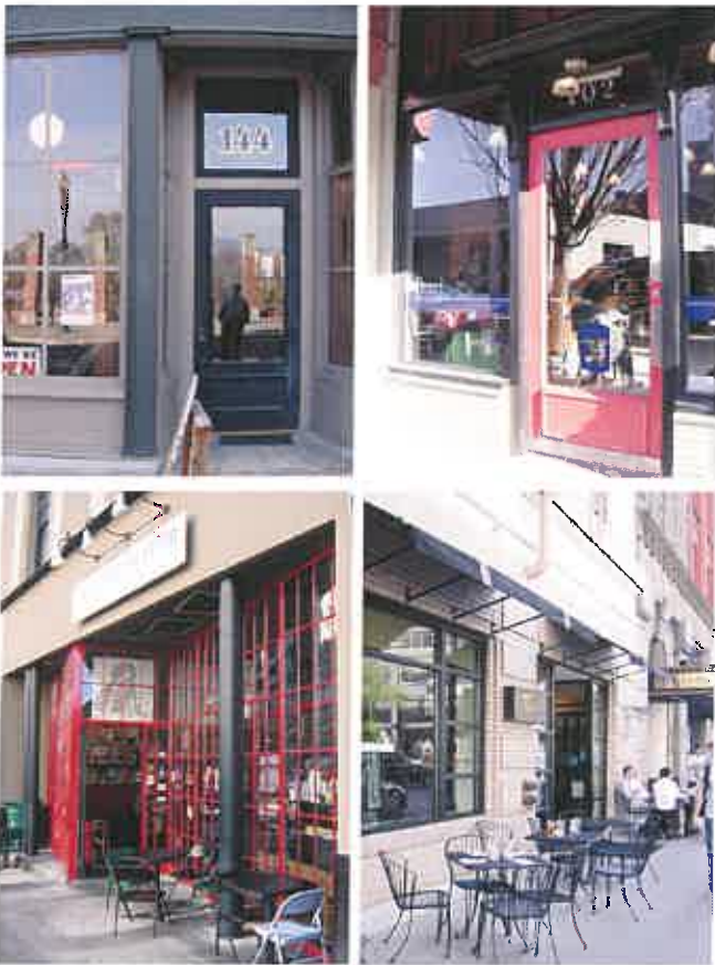
Ground-Floor Windows. [1] Using transparent windows along a minimum of 60% of the length of the ground-level street-facing facade and 60% of the overall ground-floor area provides transparency so that [2] pedestrians can see inside the building [3] Ground floor windows that incorporate vertical and horizontal elements help the ground-floor of the building relate to the scale of a pedestrian.
