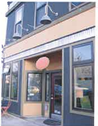
Recessed entry defined by special lighting and storefront windows and doors.
