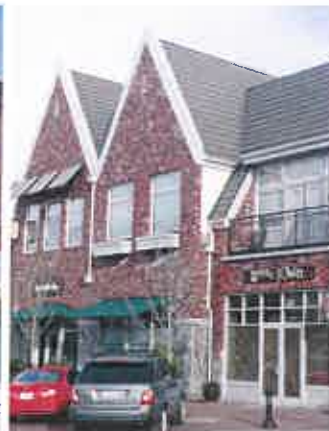
A gabled roof establishes a distinct profile and caps the facade.
