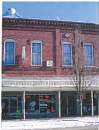
A detailed cornice and projected parapet are cap elements.
