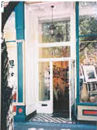
Large glass entry doors, transom windows, recessed entry bay, and pavers and colors that mark entry.
