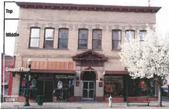
The bottom, middle, and top are distinct and readable and help to break up the building's mass.
