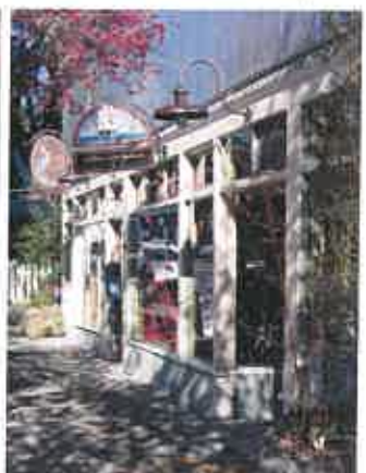
Large glass entry door, transom windows, recessed entry bay, signage, and decorative lighting.
