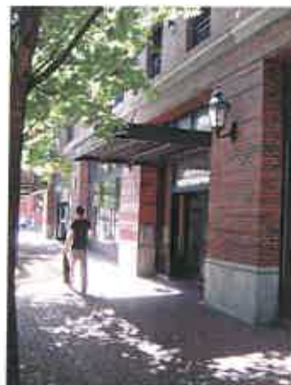
Decorative lighting, overhang, transom window, recessed entry bay, and large glass entry doors.
