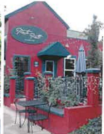
Courtyard with exterior lighting, fence, and planter boxes.
