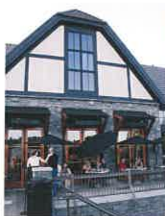
A gable roof with a hip emphasizes the top of the building.
