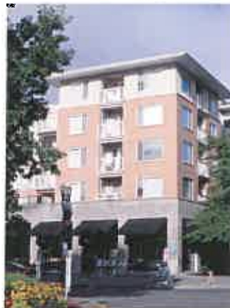
Change in color and material, vertically oriented windows signaling a change in use, and balconies distinguish the middle of the building.
