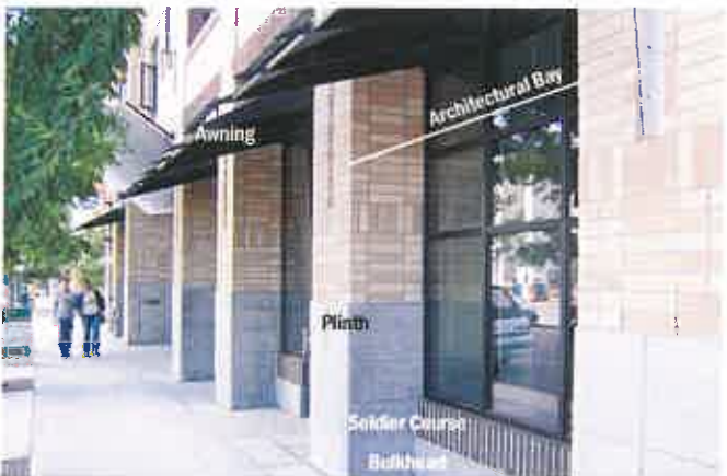
Large storefront windows, awnings, and a tall ground floor height enhance the character of the ground floor. Plinths, a projected soldier course, and the bulkhead articulate the base.
