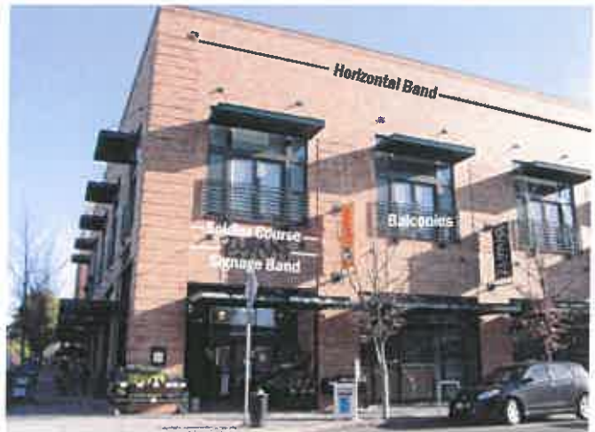
Vertically oriented windows signaling a change in use, horizontal bands, signage bands, balconies, awnings, and a brick soldier course distinguish the middle of the building from the ground floor.
