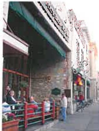
Courtyard defined within building facade with fences and planter boxes.
