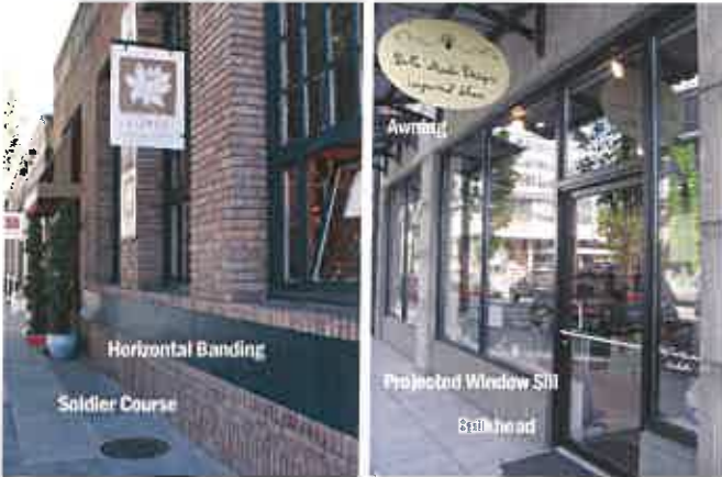
Brick soldier course defines bottom of base of ground floor and horizontal banding of a different color defines top of base.
