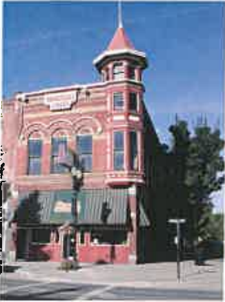
Primary entry within 25 feet of corner and prominent turret articulate gateway into downtown and provide a means of way finding.
