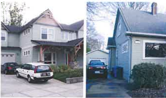
Yards. [1] The minimum front setback for detached dwellings should be 15 feet with a 4 foot setback for attached garages. [2] The minimum front setback for detached garages should be 40 feet.
