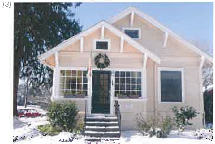
Roof Forms. [1] Roof pitches less than 6 over 12 are prohibited and roof forms will consist of more than a single large roof form [2] The primary gable shall be oriented to the street and decorated with windows, trim, or a vent [3] Roof eaves will project at a minimum 12 inches.
