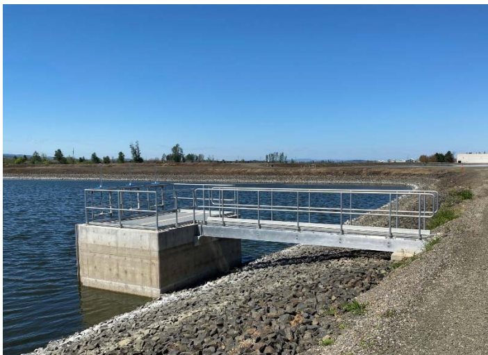
Figure 4-19 | Lagoon Cell 4 Outlet Control Structure
