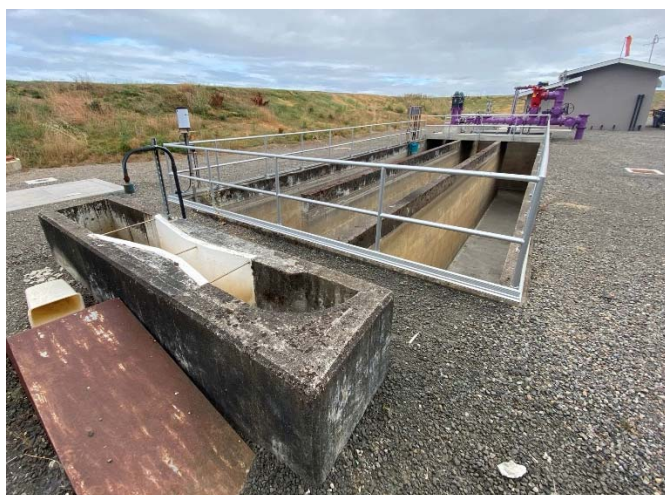
Figure 4-20 | Chlorine Contact Chamber & Parshall Flume
