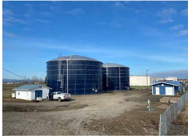
Figure 4-13 | Polk Water Treatment Plant, Pump Station & Reservoirs
