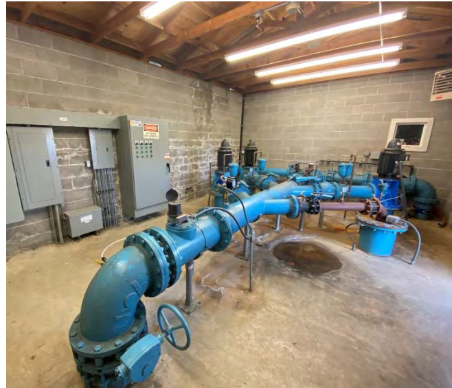
Figure 4-16 | South Water Treatment Plant
