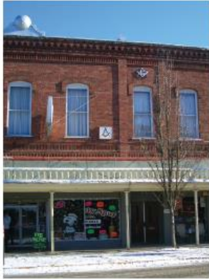
A detailed cornice and projected parapet are cap elements.
