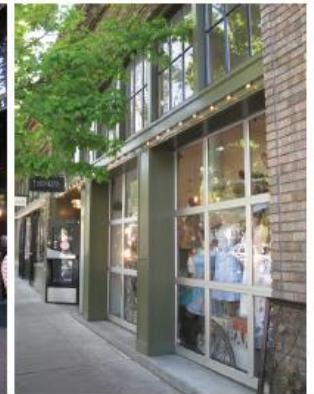
Large glass entry door, large windows, transom windows, columns, and pedestrian oriented signage.
