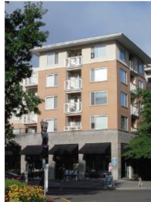
Change in color and material, vertically oriented windows signaling a change in use, and balconies distinguish the middle of the building.
