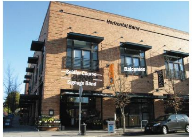
Vertically oriented windows signaling a change in use, horizontal bands, signage bands, balconies, awnings, and a brick soldier course distinguish the middle of the building from the ground floor.
