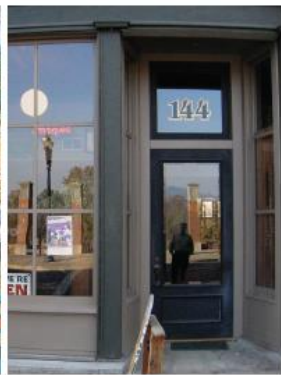
A recessed entry bay, large glass entry door, glass windows flanking the door, and columns.
