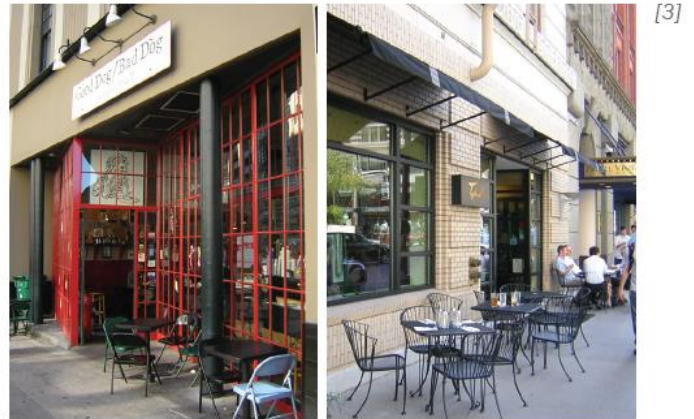
Ground-Floor Windows. [1] Using transparent windows along a minimum of 60% of the length of the ground-level street-facing facade and 60% of the overall ground-floor area provides transparency so that [2] pedestrians can see inside the building [3] Ground floor windows that incorporate vertical and horizontal elements help the ground-floor of the building relate to the scale of a pedestrian.
