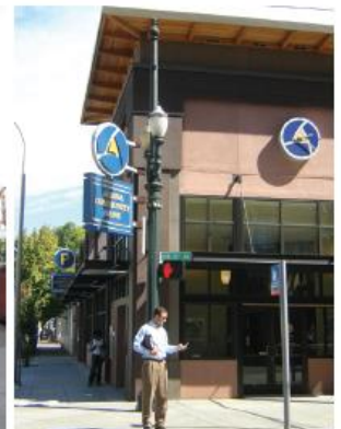
Primary entry located within 25 feet of corner, increased height at the corner and overhangs, and projecting blade sign provide a means of way finding.
