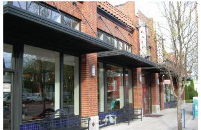
Large glass entry door, transom windows, glass windows flanking the entry door, awnings, plinths and columns, and decorative lighting. Benches provide places for passing pedestrians to pause and rest.
