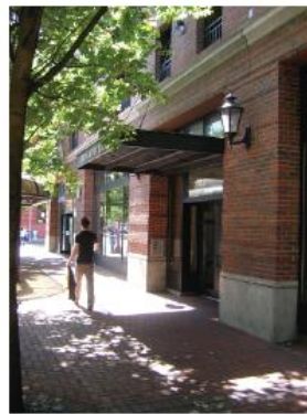
Decorative lighting, overhang, transom window, recessed entry bay, and large glass entry doors.
