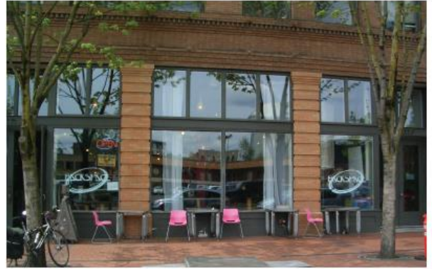
Ground floor divided into an odd number of distinct architectural bays that are 30 feet wide and defined through engaged columns. Transom windows and projected window sills are repeated in each distinct architectural bay.
