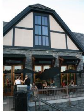
A gable roof with a hip emphasizes the top of the building.
