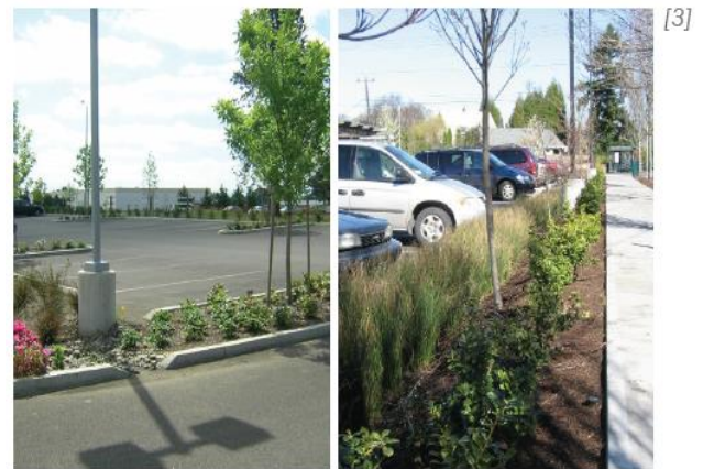
Off-Street Parking Lot Landscaping. Parking lot appearance and functionality can be improved by [1] a minimum perimeter setback of 6 feet with ground cover, shade trees, and shrubs that are a minimum of 3 feet high [2] internal landscaping strips that are a minimum of 8 feet wide [3] and stormwater detention and retention landscaping that reduces run-off while also providing a buffer between parking and pedestrians.
