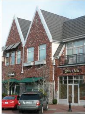
A gabled roof establishes a distinct profile and caps the facade.
