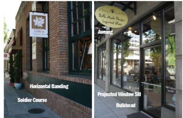
Brick soldier course defines bottom of base of ground floor and horizontal banding of a different color defines top of base.
