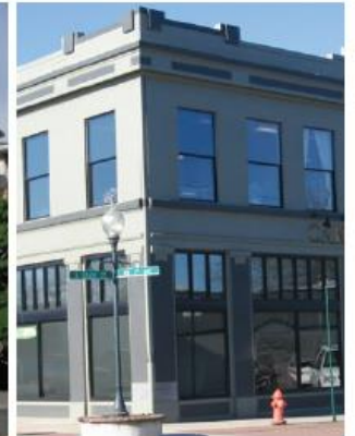
Vertically oriented windows signalling a change in use and horizontal banding distinguish the middle of the building.
