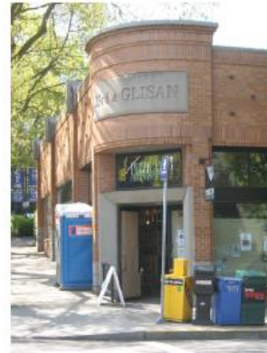
Primary entry on the corner and increased height provide public meeting space and reflects historical structures.
