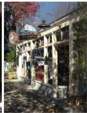
Large glass entry door, transom windows, recessed entry bay, signage, and decorative lighting.
