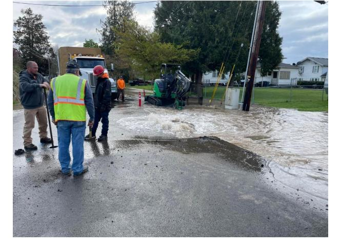
On April 4, 2024, contractors working on a sewer line replacement on C street broke through a water main, resulting in low water pressure across the city. As a precautionary measure, the city issued a boil water notice until water samples could be tested for possible contamination. All tests came back negative for contaminants. During the incident, our public works crew repaired the broken main and issued a stop worker order.
