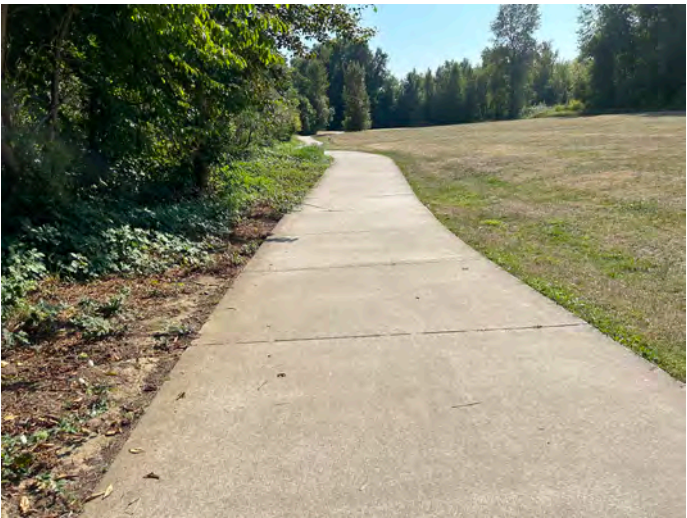
Willamette River Trail Concrete Path Connection
