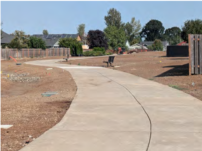
Concrete Circulation Path and Benches
