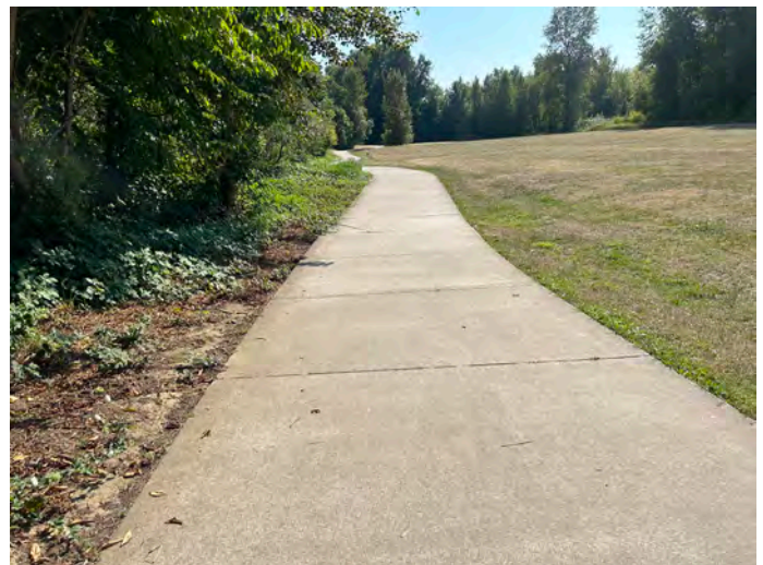
Willamette River Trail Concrete Path Connection
